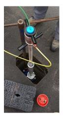
The SynthoCam H<sub>2</sub>O system has been designed for live access into potable water pipes through full bore hydrants or under pressure drillings from a vertical insertion system.
