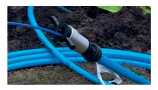
Tracing wires can be inserted end on into a PE service, through a top tee into a polyethylene main, using a through-bore hydrant or through an Elster meter box.
